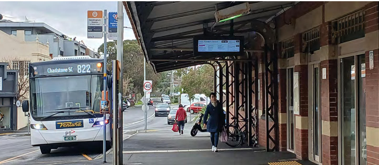
Sandringham station, a rare Melbourne example offering largely weather protected interchange between train and bus.
