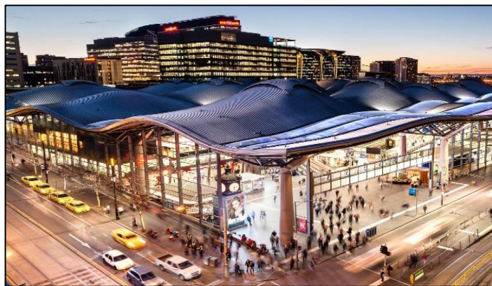
Distinctive wave form roof spanning platforms 1 to 15 between Collins & Bourke Street at Southern Cross station.
