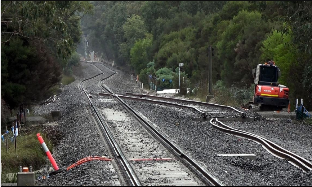
Single to Double track junction at Longwarry.
