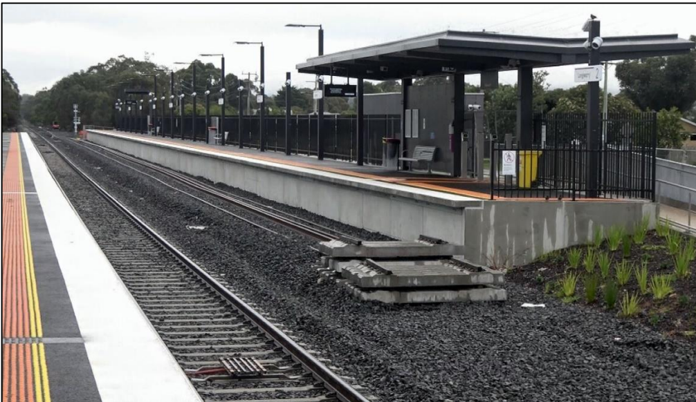
Yet to be commissioned new future second platform at Longwarry.
