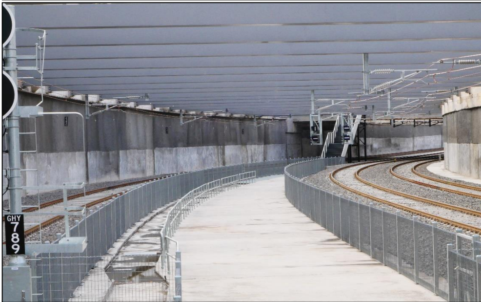
Departing the new Glen Huntly Station looking towards Caulfield in the Up direction
