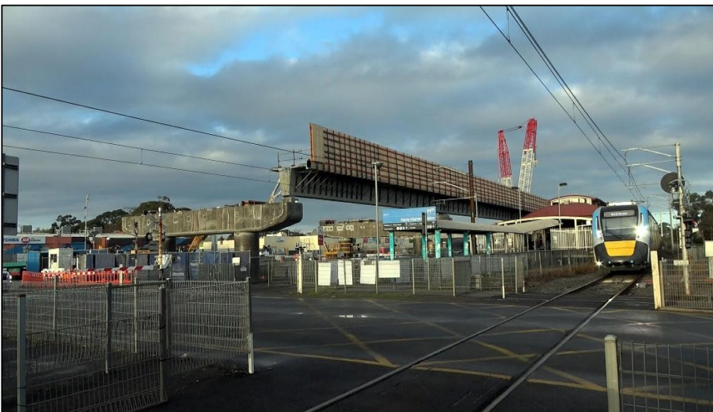
New rail over road grade separation and HCMT train at Narre Warren.
