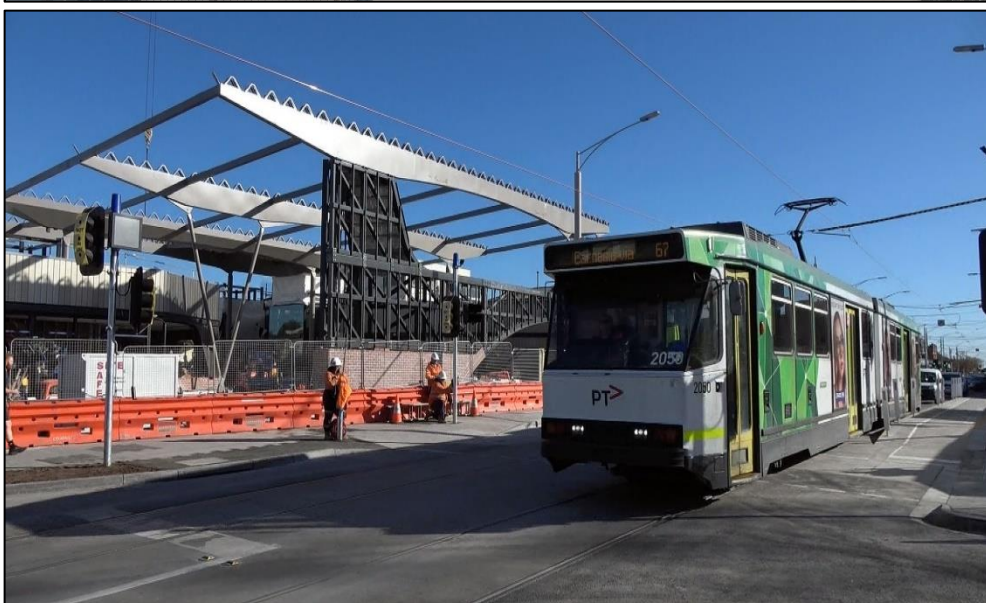
B-2 Class tram outbound on Route 67 to Carnegie passes over the new Glen Huntly station below in a three track trench.
