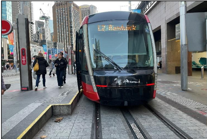
Sydney Light Rail showing between tracks power source.
