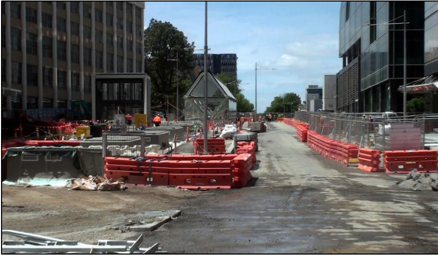
Glass entry to PARKVILLE station on Grattan Street Photo - Jonathan Scutt
