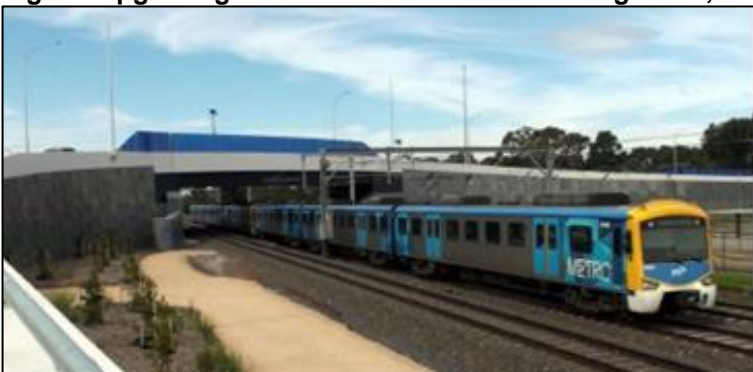
Below: Left - MTM train departing Werribee on the Up beneath a new road overpass which spans three tracks and replaces a level crossing with complex road intersections on both sides of the rail corridor. Photo – Jonathan Scutt Right – Upgrading Echuca line north of Goornong June, 2022 for 100 km/h DMU line speed. Photo – David Hardy
