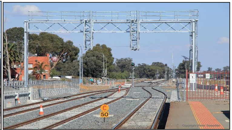
Above and below – Four photos of the new crossing loop at Murchison East with a centre crossover so a goods train can be put away whilst two passenger trains also cross.. Photos- courtesy of Rail Projects Victoria.
