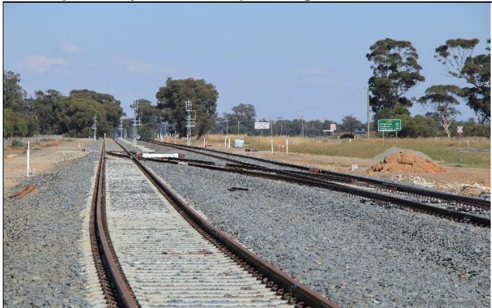
Above and below – Four photos of the new crossing loop at Murchison East with a centre crossover so a goods train can be put away whilst two passenger trains also cross.. Photos- courtesy of Rail Projects Victoria.
