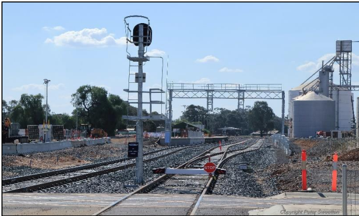
Above and below – Four photos of the new crossing loop at Murchison East with a centre crossover so a goods train can be put away whilst two passenger trains also cross.. Photos- courtesy of Rail Projects Victoria.
